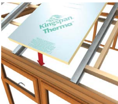
Install external insulation
