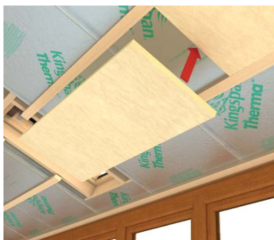
Install insulation between batten
