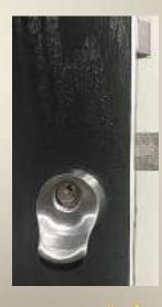
As an additional benefit, because of the absence of a lever handle, a door fitted with a Heritage Autolock prevents 'follow-in' as once the hooks automatically engage, access can only be made by a second person by a quarter turn of the key to release the hooks.
